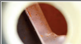
A glance underneath the tank cap gives an idea about the amount of rust inside the tank
